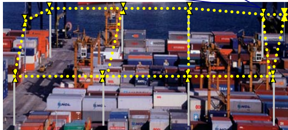
Figure 3: RELAYER™ ad hoc RF network installed around the yard communicates to the monitoring station all quiescent signals from redundant ZONER™ devices placed inside each container. Tampering and exceptions are reported in real-time to local or destination custom authorities and others with need-to-know. Detailed data is also stored by an Independent Monitoring Agency.
